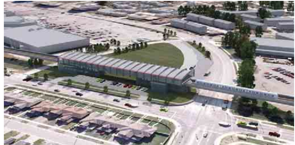
Future Malvern Station
