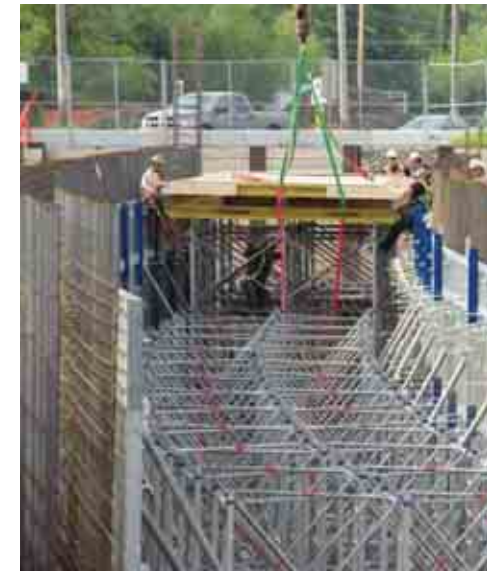
The concrete tunnel is poured and then the surface is reinstated.
